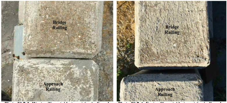
Photo 58.7-3: West railing at Abutment 6 misaligned transversely 1 inch to the west
